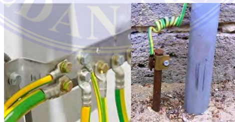
Gambar 2.5 Sistem Grounding
