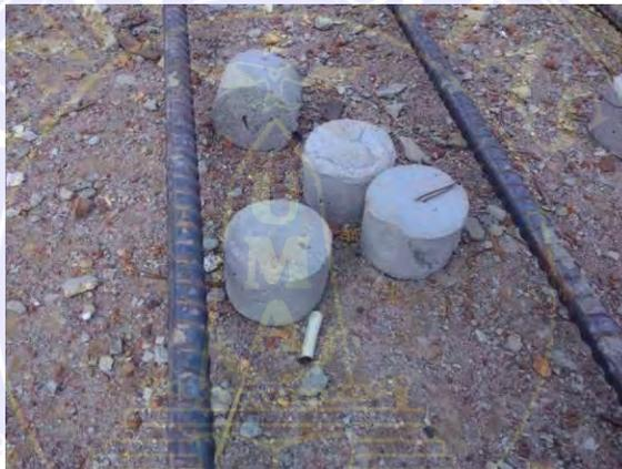
Gambar 4.21 Beton *Decking*
