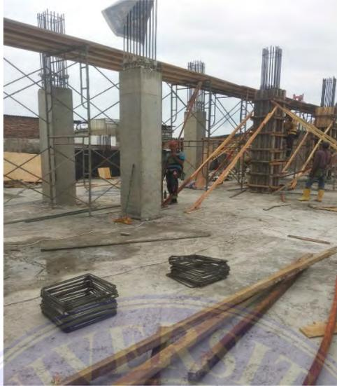
Gambar 5.5 Pelepasan Bekisting
