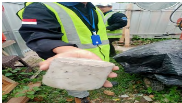
Gambar 2.2.7 Beton Decking
