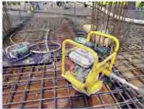
Gambar 3.3 Beton Vibrator
