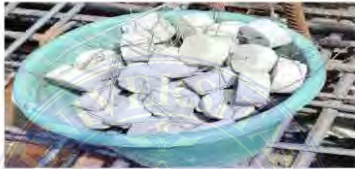
Gambar 3.20 Beton Decking
