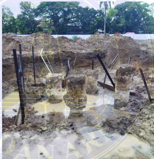
Gambar 4.12 Pondasi Bore pile
