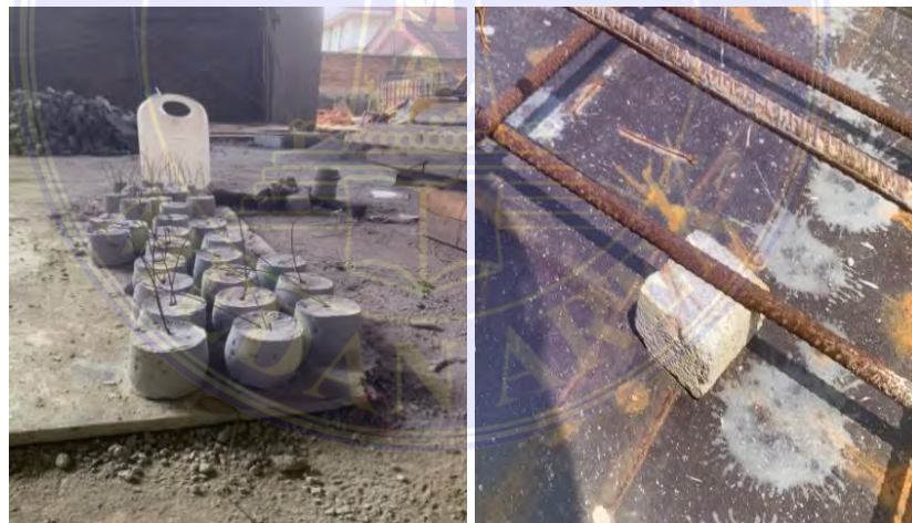
Gambar 3.37 Beton Decking
