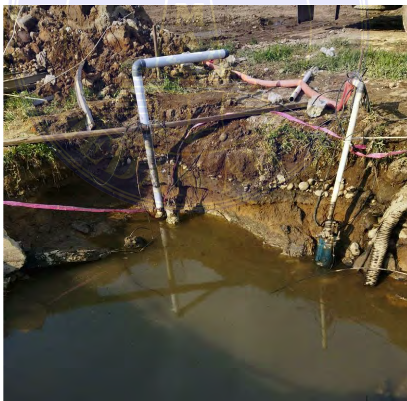
Gambar. Proses Dewatering
