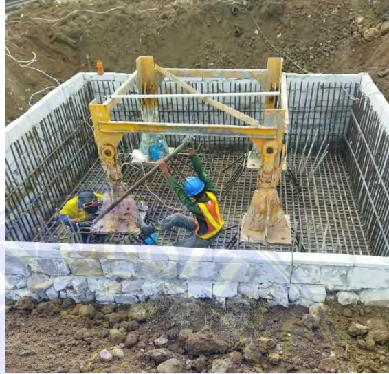
Gambar 4.16 Proses setting Anchor
