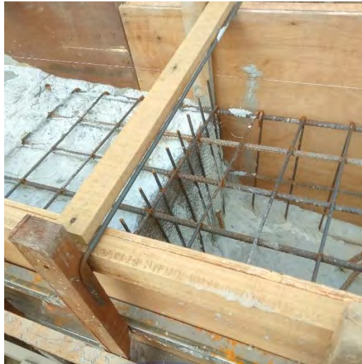
Gambar 4.7 Pengecoran Capping Beam
