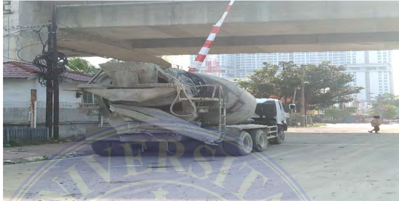
Gambar 3.10 Truck Mixer Beton
