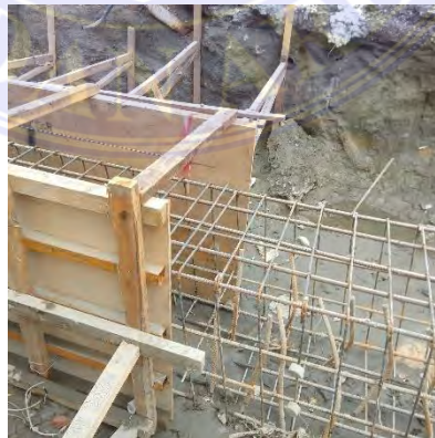
Gambar 3.9 Bekisting Capping Beam
