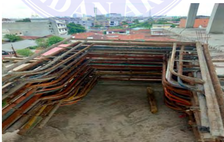
Gambar 3.1.27 Scaffolding Sumber : Lampiran Lapangan
