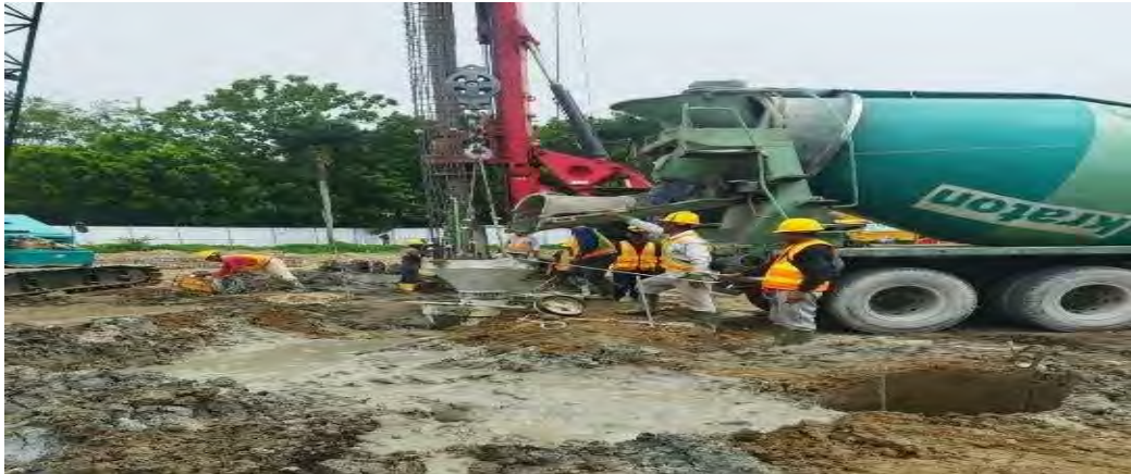
Gambar 13 Truck Mixer Beton
