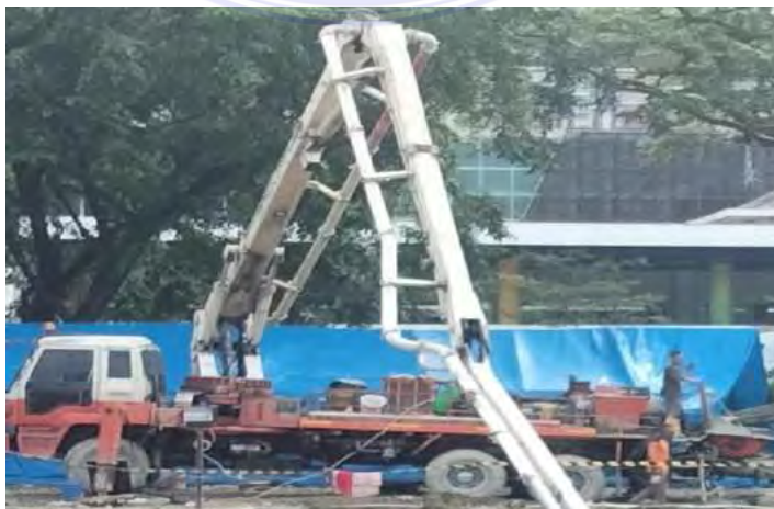
Gambar 3.11 Pompa Beton/ Concrete Pump Truck Sumber : Data Lapangan
