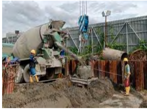
Gambar 3.1.9 Truck Mixer Beton
