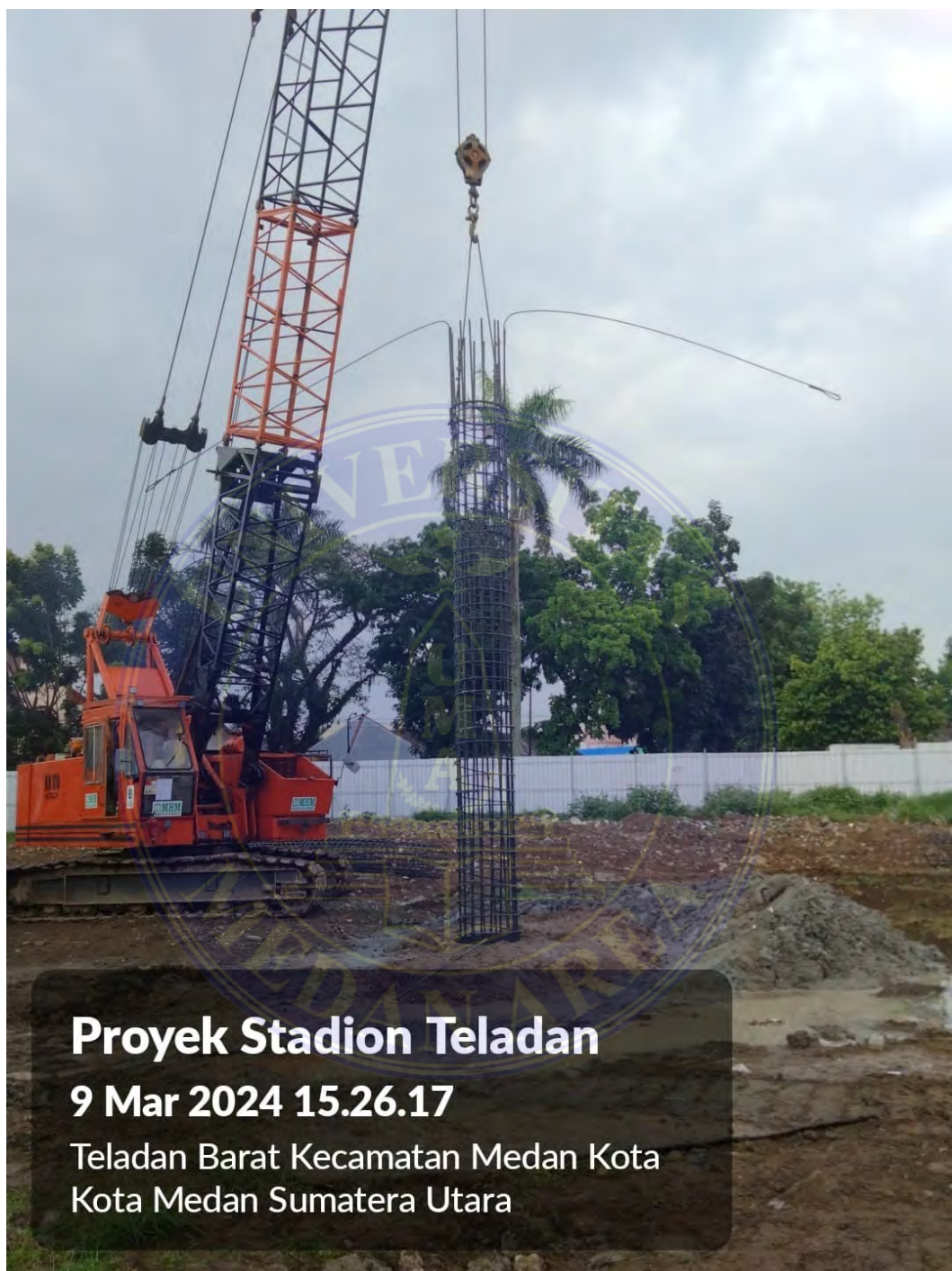
Gambar: Install besi
