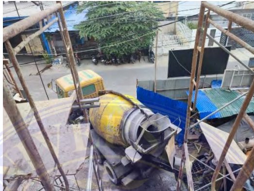
Gambar 3. 10 Truck Mixer Beton
