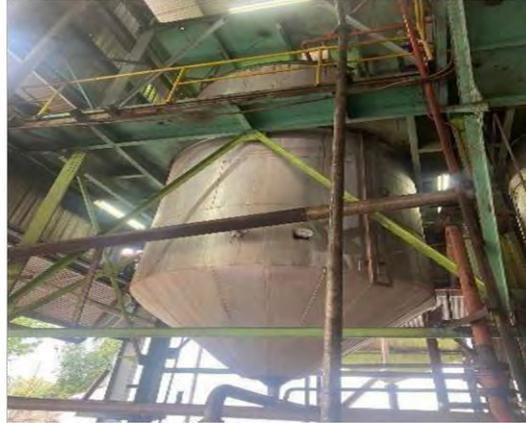
Gambar 3.19 Sludge Tank
