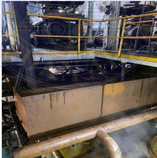
Gambar 3.11 Oil Gutter
