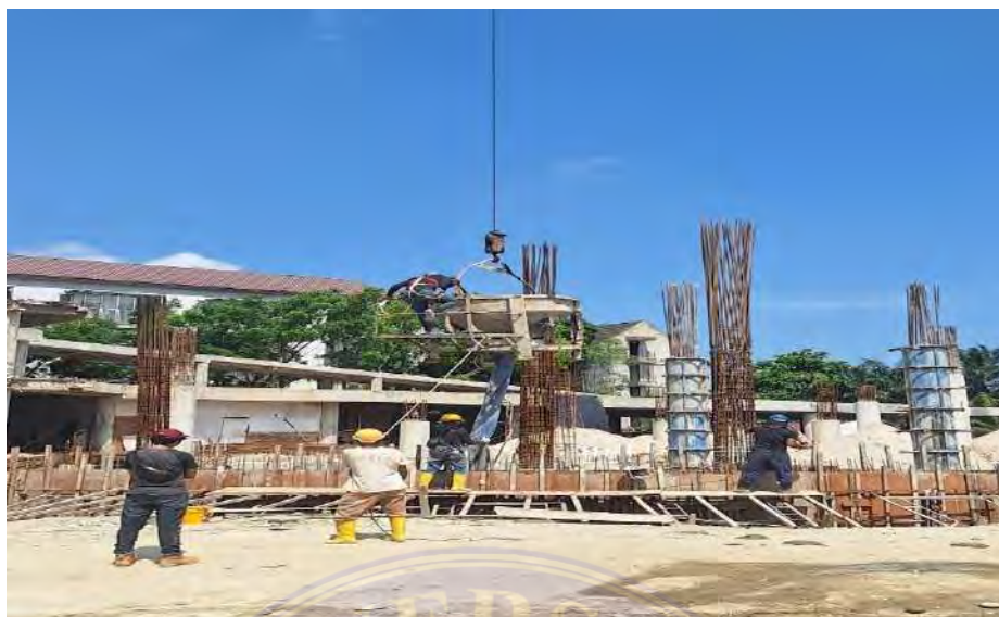
Gambar 5. Pengecoran Dinding Penahan Tanah
