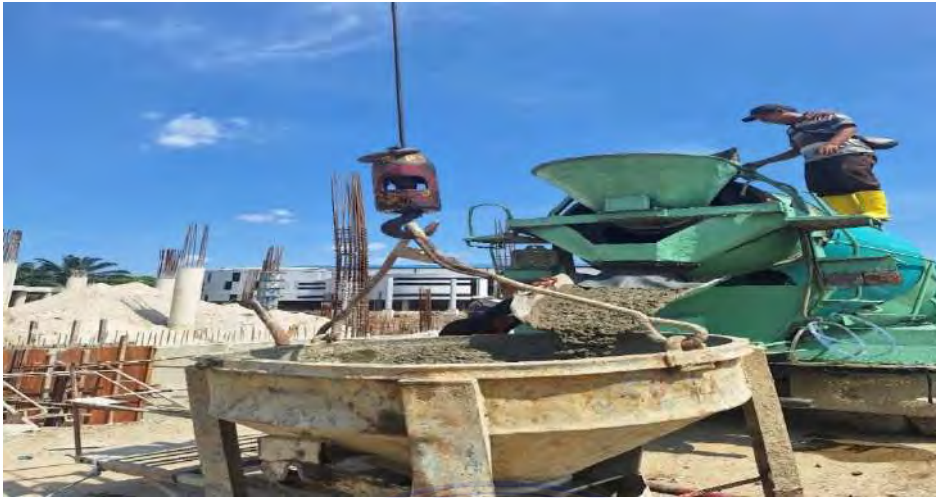
Gambar 4.10. Beton ready mix ke concrete bucket ,
