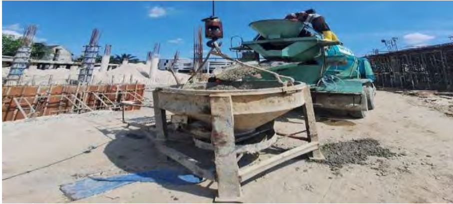
Gambar 3.15 Concrete Bucket ,
