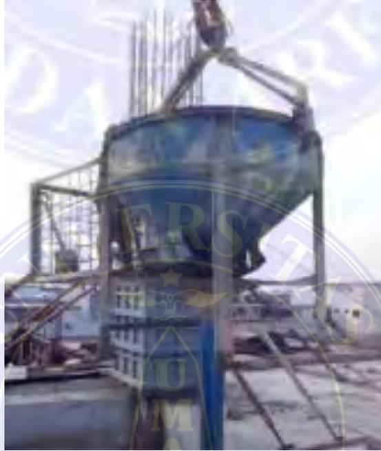
Gambar 4.30 *Concrete Bucket*
