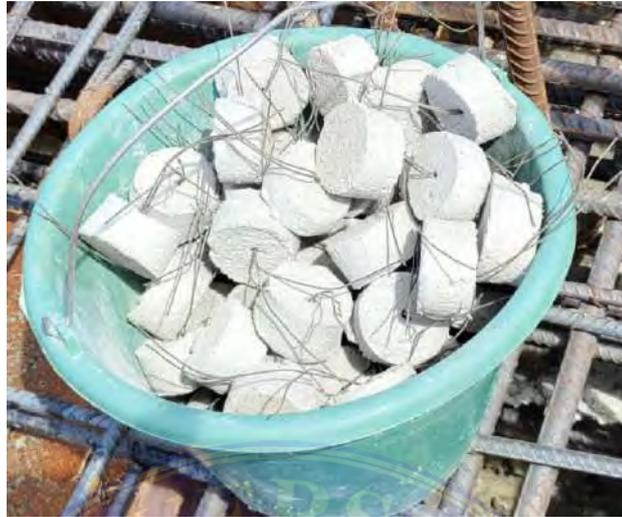
Gambar 4.19 Beton *Decking*
