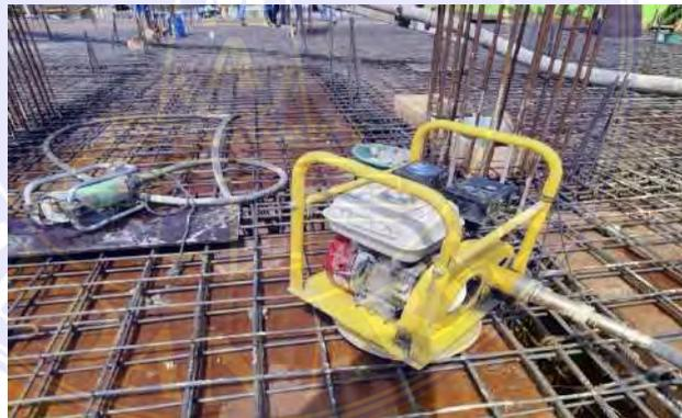
Gambar 4.3 Beton *Vibrator*
