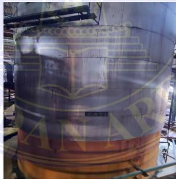
**Gambar 3. 37 Continuous Settling Tank**
