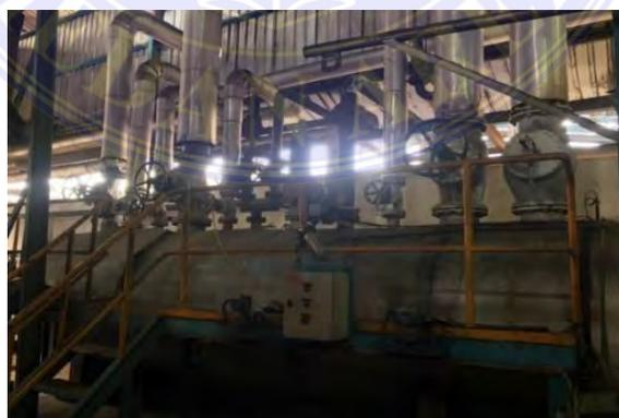
**Gambar 3. 58 Back Pressure Vessel (BPV)**
