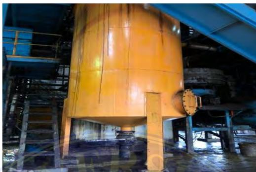
**Gambar 3. 34 Sand Trap Tank**
