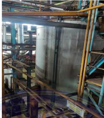
**Gambar 3. 38 Sludge Tank**
