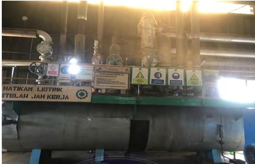
Gambar 3.45. *Back Pressure Vessel*
