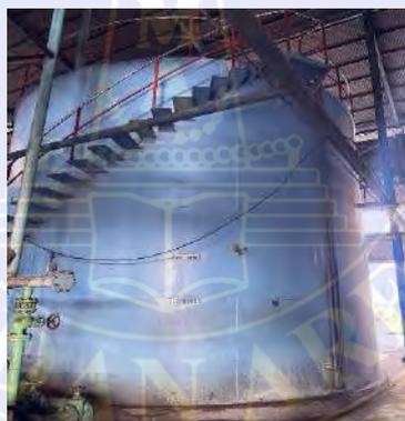
**Gambar 3. 41 Feed Water Tank**
