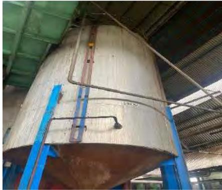
**Gambar 3. 21 Sludge Tank**
