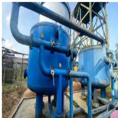
**Gambar 3. 36 Pressure Sand Filter**
