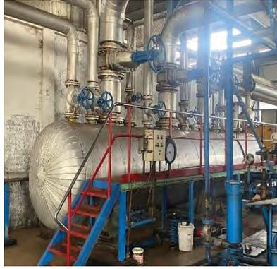
**Gambar 3. 35 Back Pressure Vessel (BPV)**
