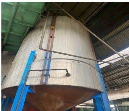
**Gambar 3. 23 Sludge Tank**
