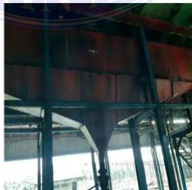
**Gambar 3. 15 Sand Trap Tank**
