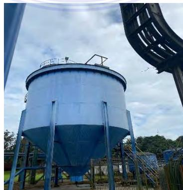
**Gambar 3. 36 Water Clarifier Tank**
