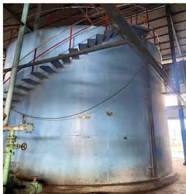
**Gambar 3. 43 Feed Water Tank**
