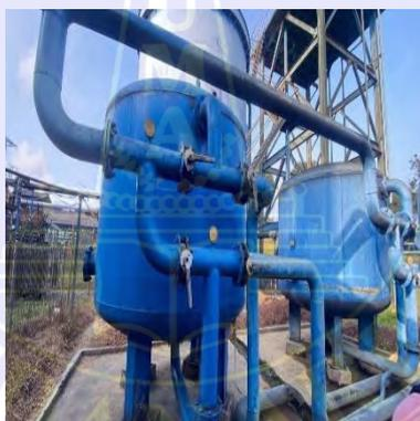
**Gambar 3. 38 Pressure Sand Filter**
