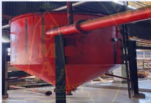
**Gambar 3.32 Sand Trap Tank**
