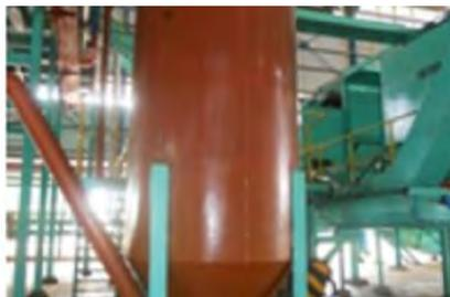
**Gambar 3. 35. Sand trap tank**
