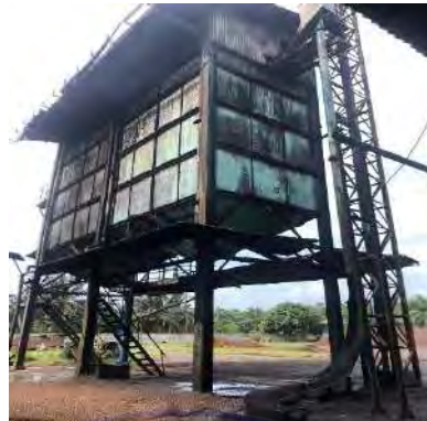
Gambar 3. 31 Kernel Bunker
