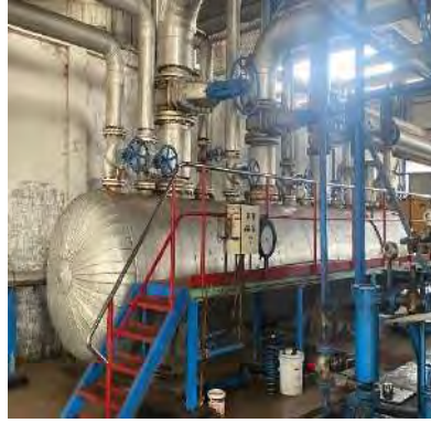
Gambar 3. 35 Back Pressure Vessel (BPV)
