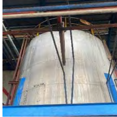
Gambar 3. 20 Wet Oil Tank
