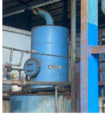
Gambar 3. 41 Degasifer Tank
