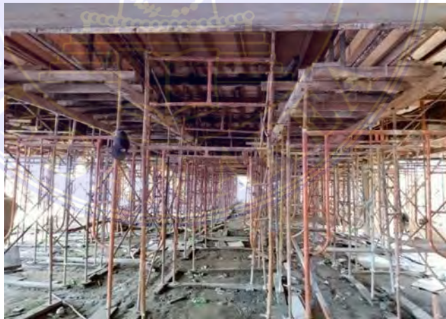
Gambar 4.2 Pemasangan Scaffolding.
