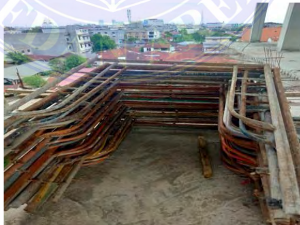
Gambar 3.19 Scaffolding Sumber: Data Lapangan
