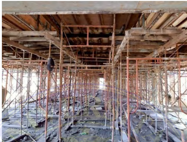
Gambar 1 Pemasangan Scaffolding.
