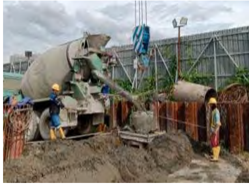
Gambar 3.1.9 Truck Mixer Beton
