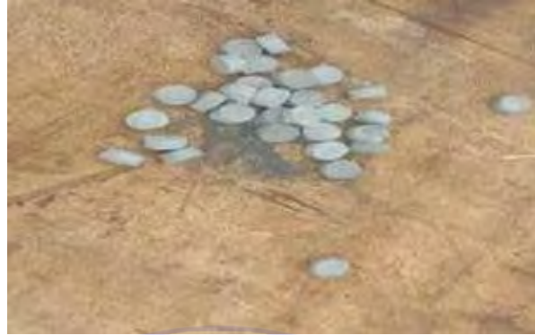
Gambar 3.2.12 Beton Decking
