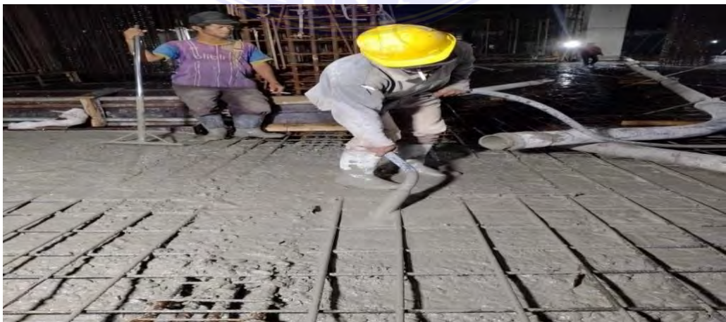
Gambar 3.12 Concrete Vibratrition
