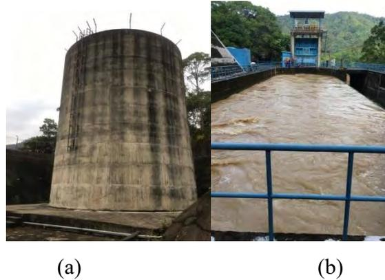
Gambar 3.6. (a). Surge tank, (b). Head tank
