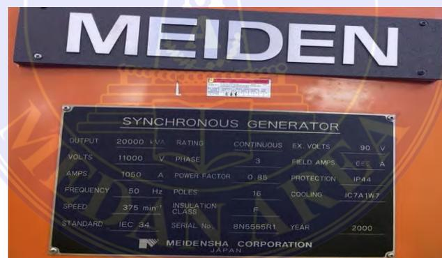
Gambar 3.10. Name plate generator PS2
