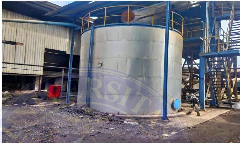
Gambar 3.51. *Feed Water Tank*
