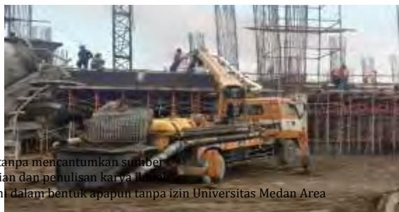
Gambar 2.3 Concrete Pump
