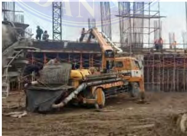
Gambar 4. 2 *Concrete Pump*
