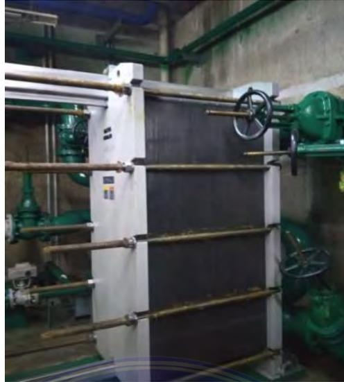
Gambar 3.26. Heat Exchanger
