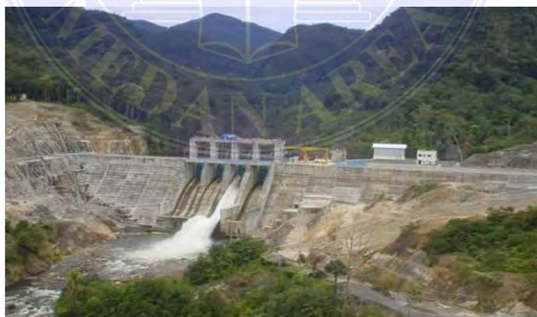
Gambar 3.3. Spillway ULPLTA Sipansihaporas
