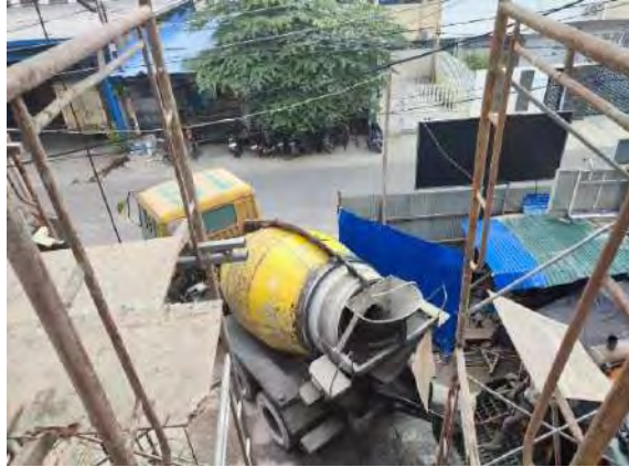
Gambar 3.10 Truck Mixer Beton
