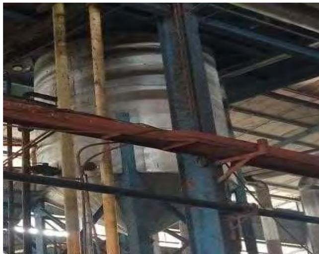
Gambar 3.23. *Sand Trap Tank*
