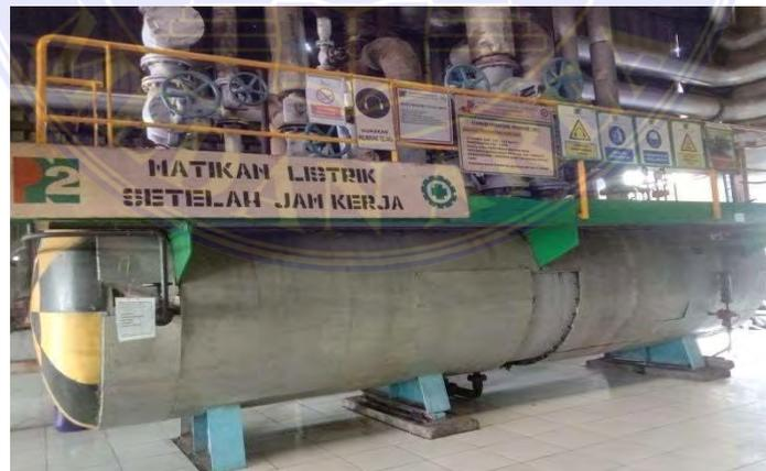
Gambar 3.55. *Back Pressure Vessel*.
