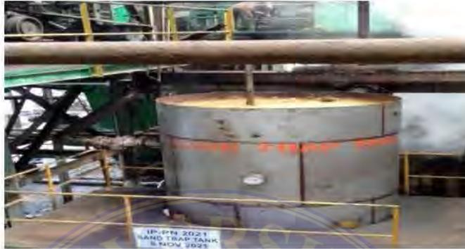
Gambar 3.13. *Sand Trap Tank*
