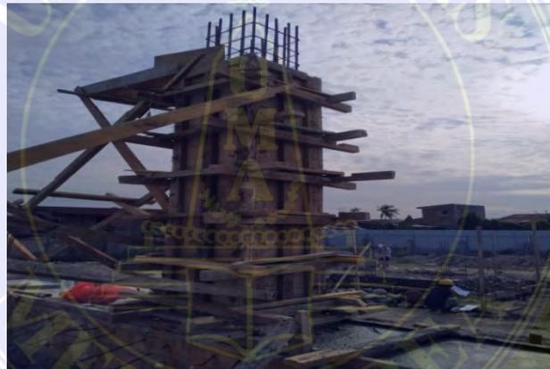
Gambar 3.6 Bekisting (Kolom)
