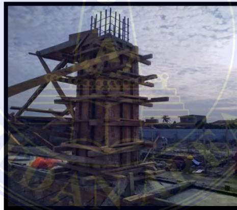
Gambar 4.6 Bekisting Kolom
