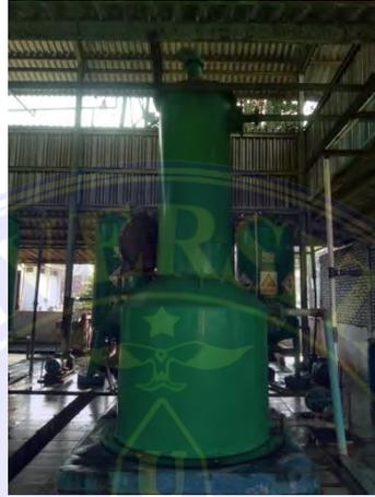
Gambar 3.29. *Degasifire Tank*
