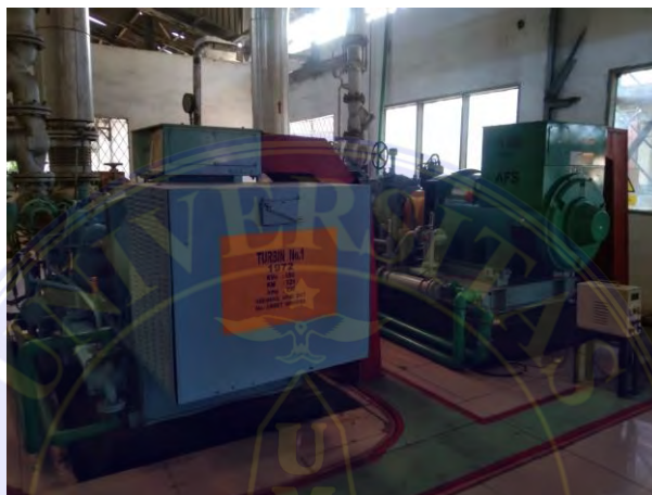
Gambar 3.26. Turbin Uap
