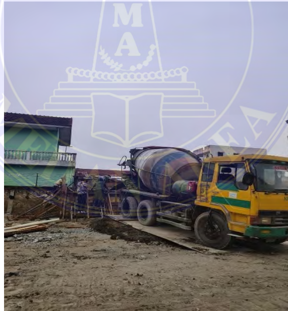
Gambar 2.6 Truck Mixer Sumber: Data Lapangan 2023
