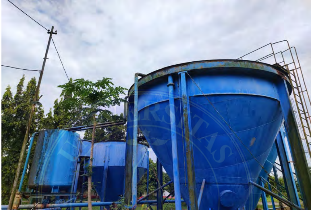
Gambar 3. 52 Clarifier Tank
