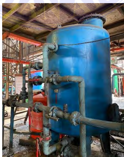
Gambar 3. 32 Anion Exchanger
