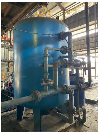
Gambar 3. 31 Katiom Exchanger
