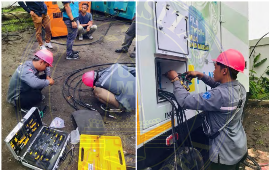
Gambar 5. Instalasi ups
