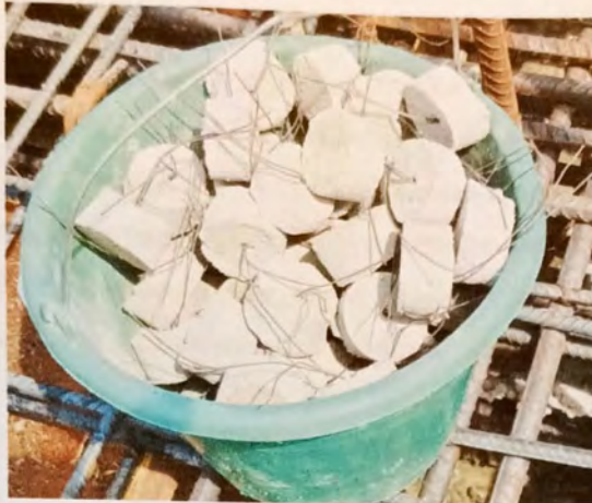
Gambar 3.20 Beton Decking
