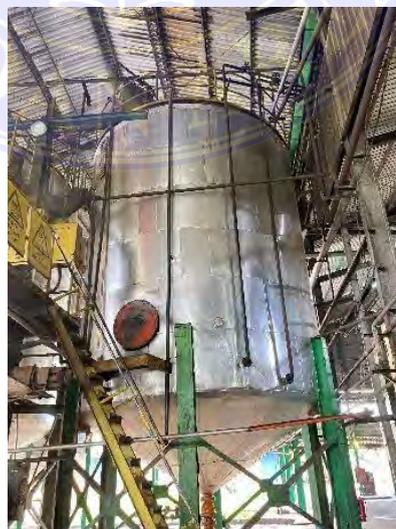
**Gambar 3.16 Continuous Settling Tank (CST)**
