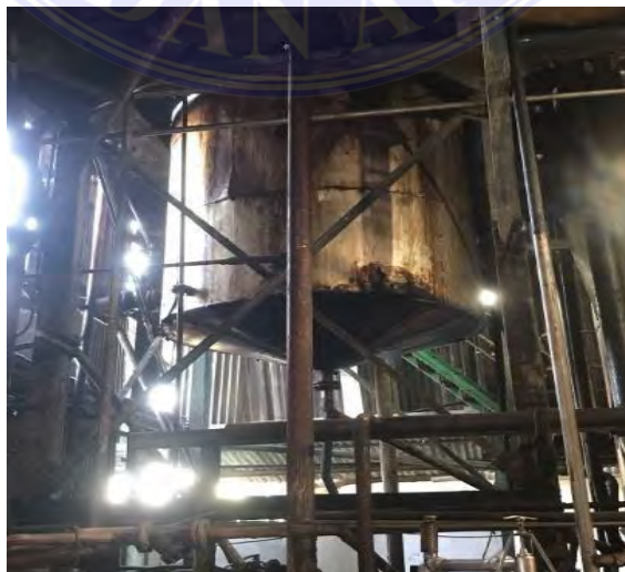
Gambar 3. 11 Bak Reverse Osmosis
