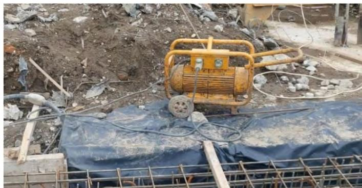
Gambar 3.2 *Vibrator Concrete*
