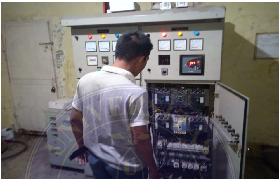
Gambar 5.1: panel kontrol kapasitor bank
