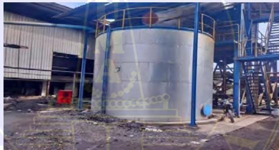
Gambar 3. 50. Feed Water Tank
