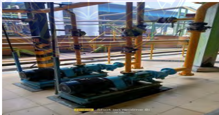
Gambar 3.6. Oil Pump final Transfer
