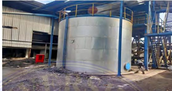
Gambar 3. 50. Feed Water Tank
