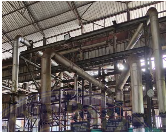
Gambar 3. 60 Back Pressure Vessel (BPV)
