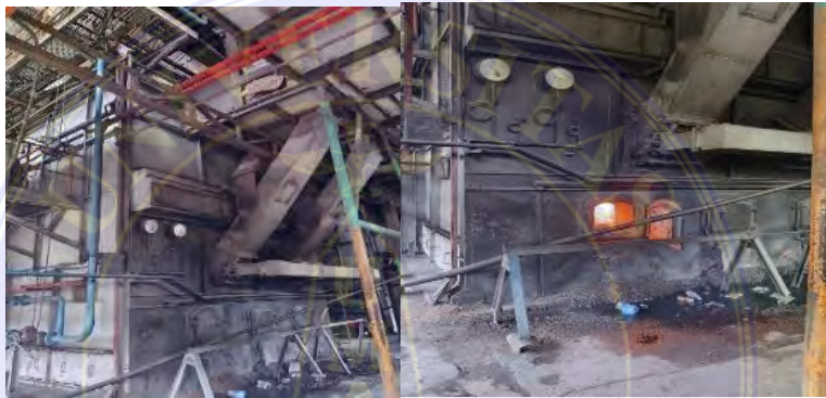
Gambar 3. 57 Ketel Uap ( Boiler )
