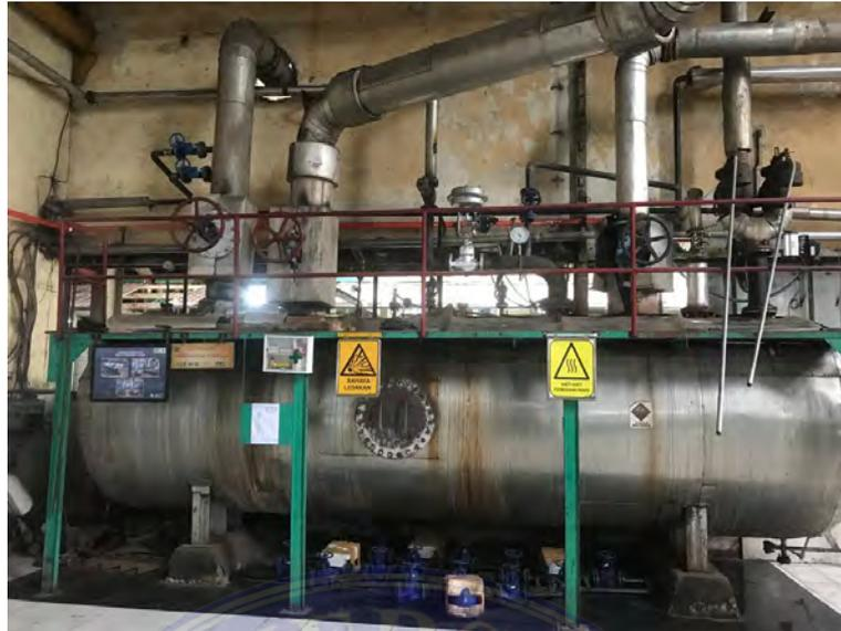
Gambar 3.58. *Back Pressure Vessel*
