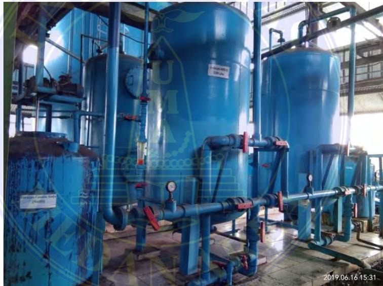
Gambar 3.55. *Anion Tank* dan *Kation Tank*
